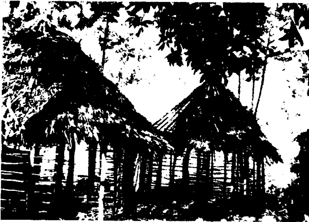
Building the Kamiti post
